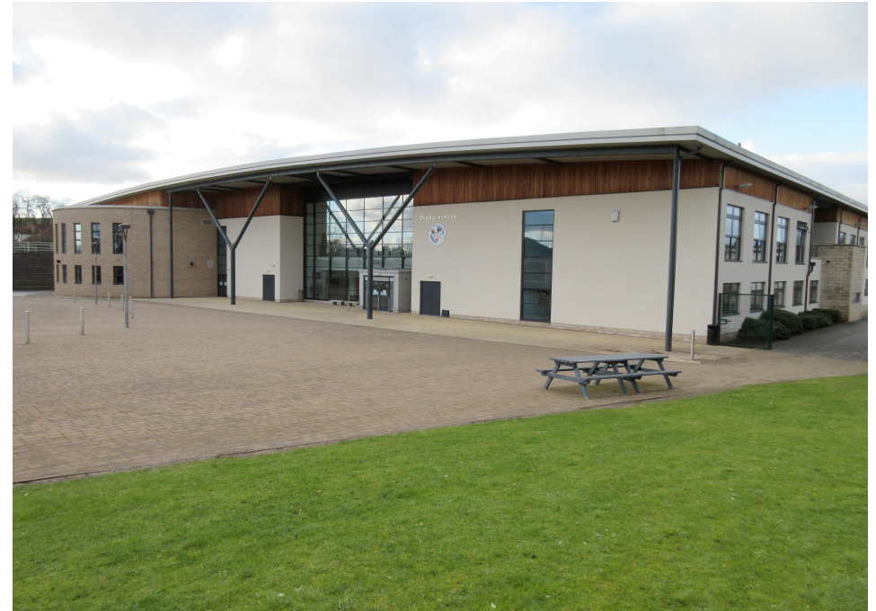
Douglas Academy, Milngavie – New Building.
